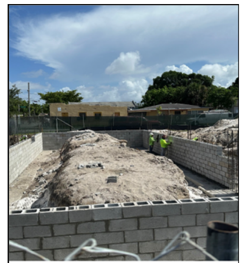
Stem Wall and Poured Foundation – Site G
