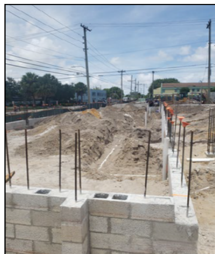
Plumbing Rough-in Site A Building B
